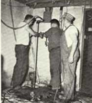
Frank Whitfield, John Bowers and George Gay finished a plumbing job.
