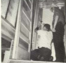
Greg Thompson and Clair Wilson hung a door on the entrance to the basement.
